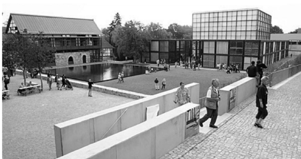
Figure 4. The landmark Hanover Expo is used as a church and has a variety of exhibition halls, Source: http://www.newsjoy.or.kr/news/articleView.html?idxno=14746
